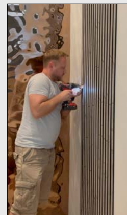
When installing without adhesive, 8 to 10 screws are recommended.
