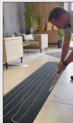
Apply assembly adhesive.
